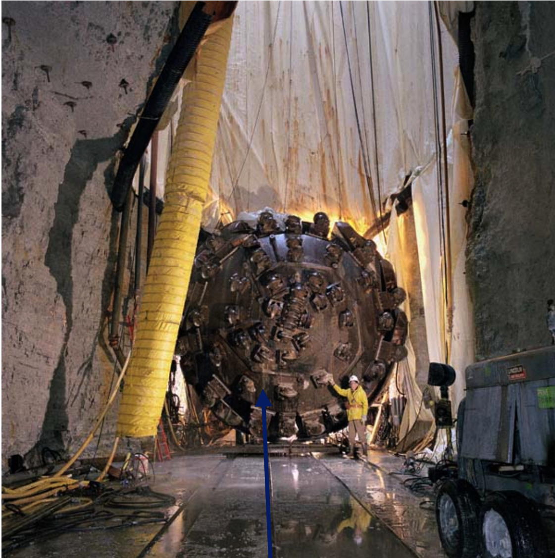
tunnel boring machine
